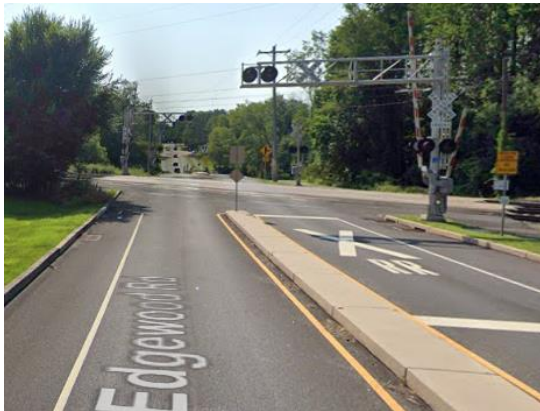
Center Lane Concrete Island
