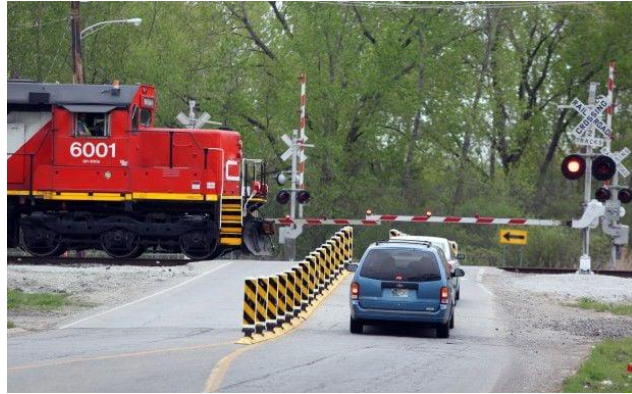
Center Lane Delineator Barriers
