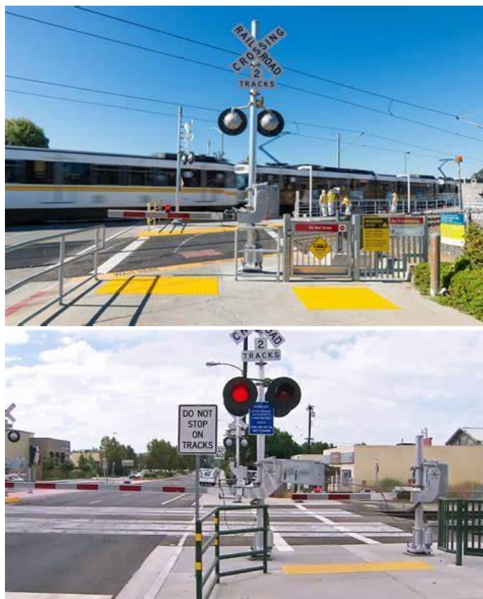
Figure 5-13. Examples of Pedestrian Grates and Sidewalks
