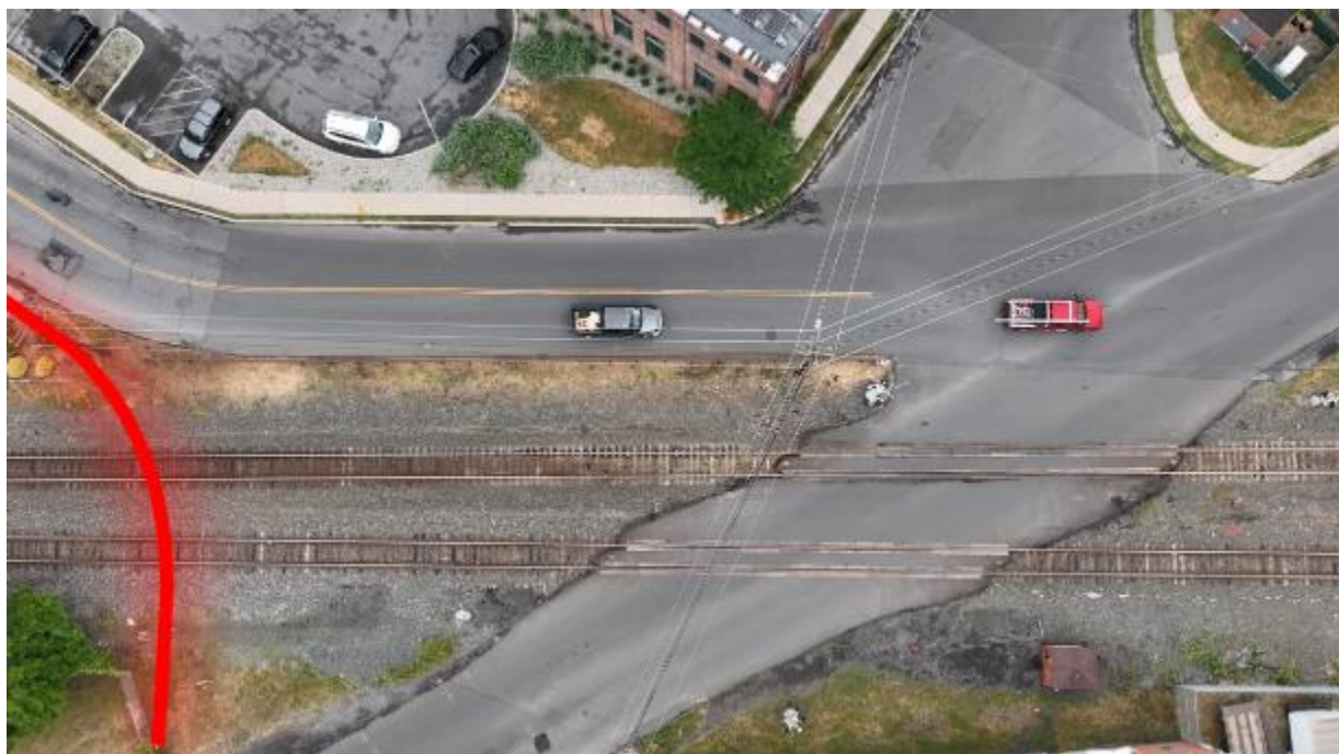
Figure 3-1. Pedestrian Pathway at Foxhall Avenue
