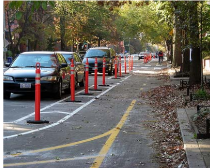
Flexible bollards can delineate a path along the Elementary School driveway
