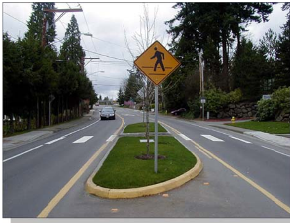
Image 7: Simple engineering measures such as pedestrian refuges can improve real and perceived safety. Source: Alta Planning + Design
