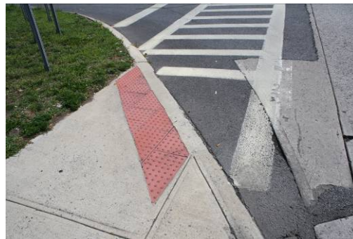
Detectible warning surface at Albany Avenue and I-587 intersection
