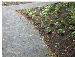
COMPACTED CRUSHED STONE CONNECTOR
