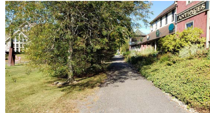
Along some sections of the trail adjacent trees will need to be pruned to provide the required trail width up to a required vertical clearance of 9'. (Empire State Trail Design Guide).
