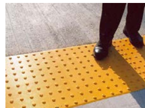
DETECTABLE WARNING STRIP
