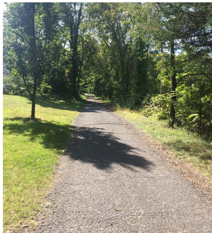
Some sections of the trail are wide enough to consider trail amenities in these locations.
