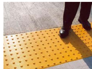
DETECTABLE WARNING STRIP
