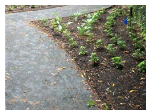
COMPACTED CRUSHED STONE CONNECTOR
