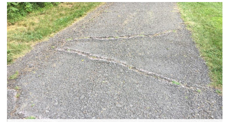
Tree roots protruding through trail
