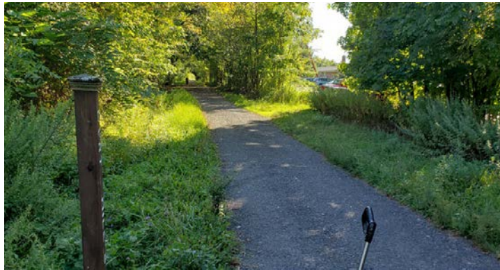
Some existing paved portions of the WVRT are less than the 8' minimum.
