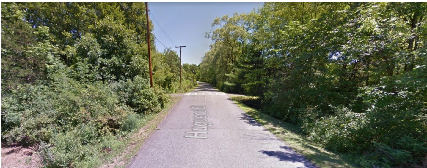
Huguenot Street at WVRT looking East
