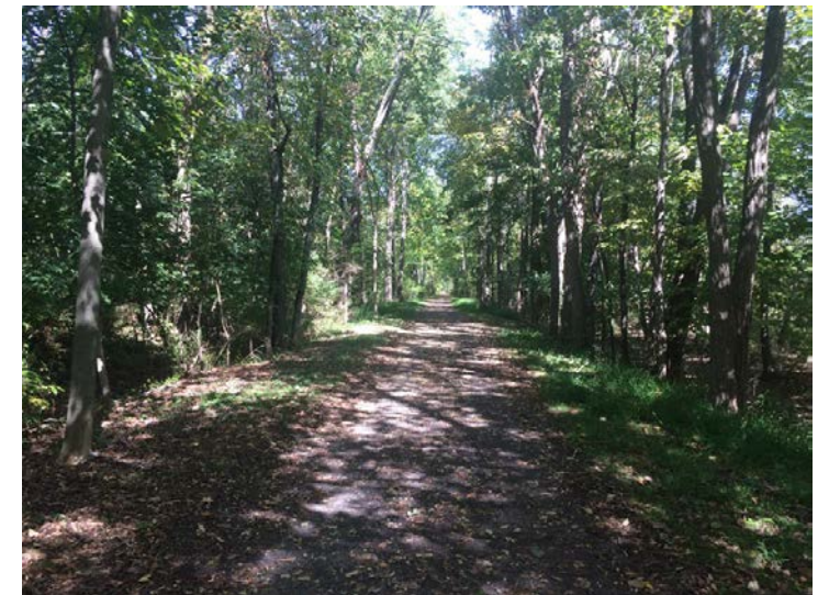
Most sections of the trail are wide enough to accommodate a 10’ minimum width with 2’ shoulders on each side.
