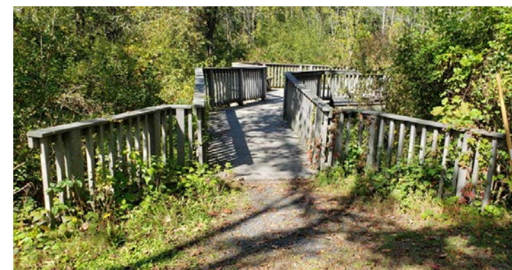
There are several viewing opportunities along the trail that can be formalized similar to this overlook.
