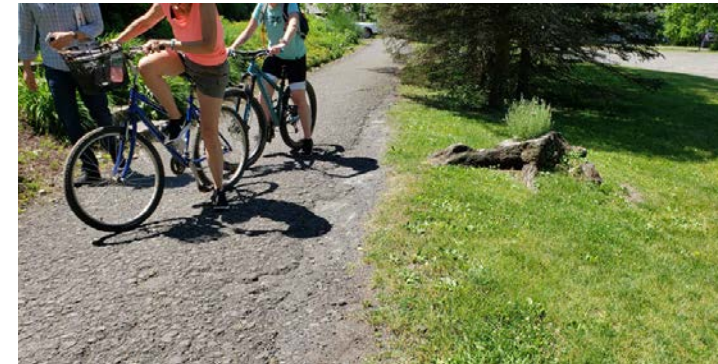
Broken and deteriorated asphalt results in rough and uneven pavement.
