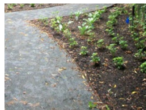
COMPACTED CRUSHED STONE CONNECTOR
