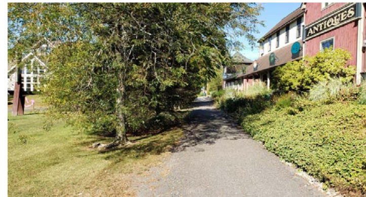
Along some sections of the trail adjacent trees will need to be pruned to provide the required trail width up to a required vertical clearance of 9’. (Empire State Trail Design Guide).
