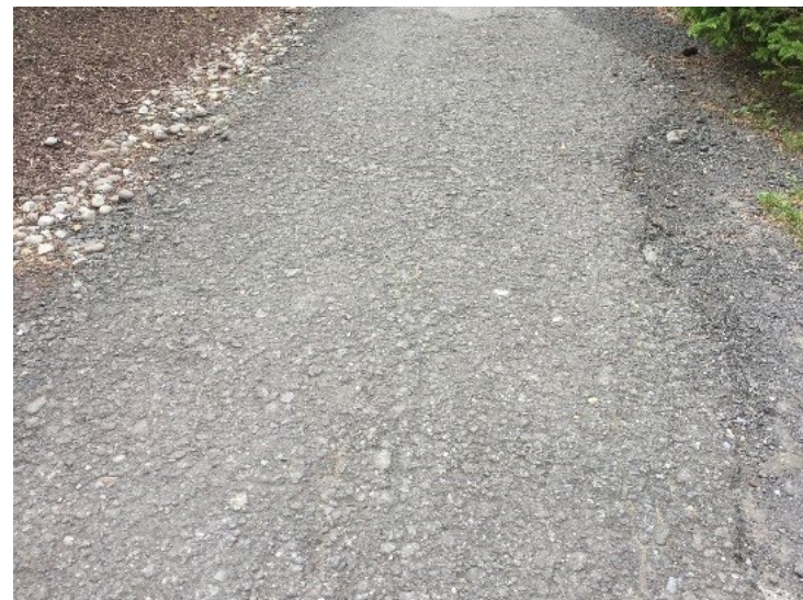
Old asphalt near Main Street
