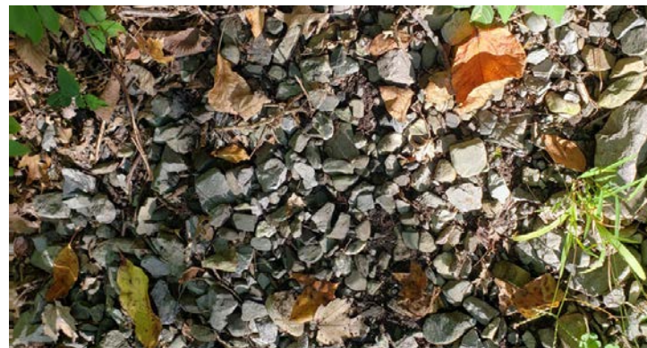
Removing the trail surface down to the ballast will allow the trail to be widened and the ballast to serve as a subbase for the new trail surface.
