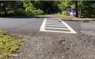
The sidewalk along the south side of North Front Street is in poor condition and does not have a smooth transition where it meets the trail. Sidewalk ends here and does not extend further towards the east.
