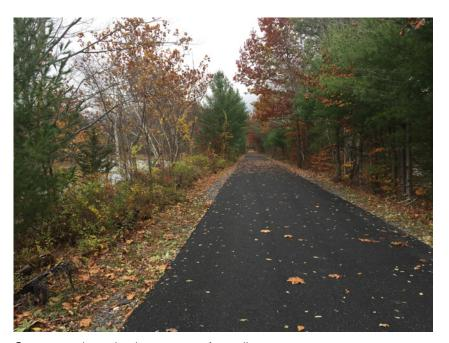
Compacted crushed aggragate for trail use.
