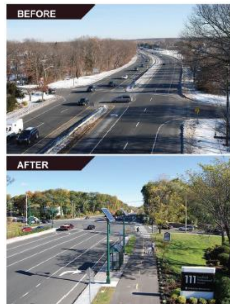
In this section of Route 347, a bicycle/pedestrian path has been added to allow pedestrians and bicyclists to travel safely and easily down the road.
