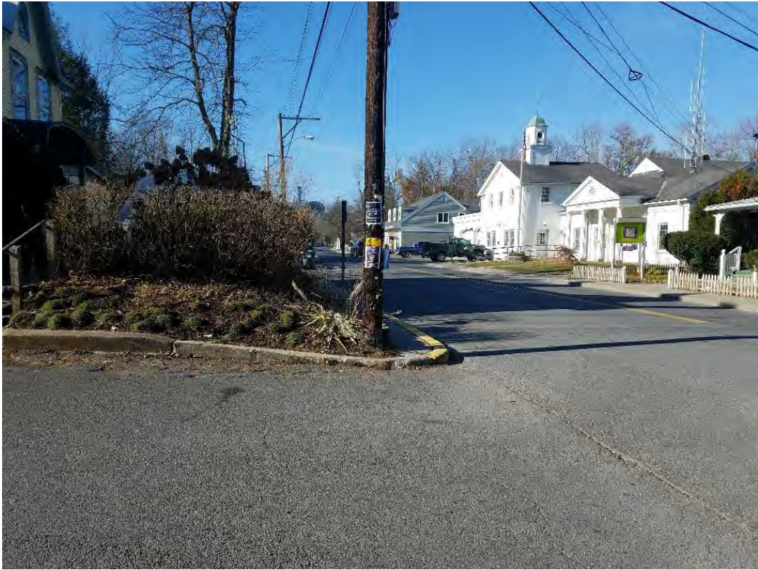
Photo 7: Shrubs obstructing sight lines at Nehrer Street.
