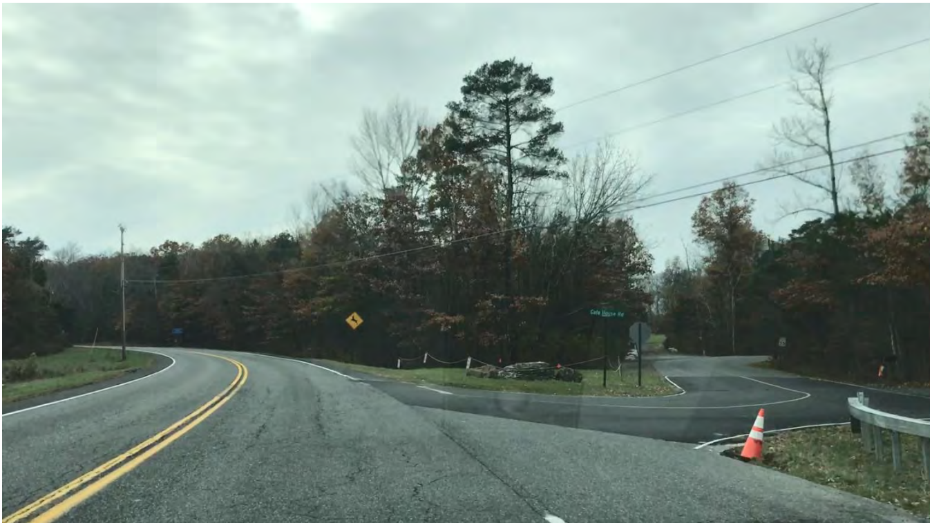
Photo 10: Tight right turn radius at Gate House Road (in vicinity of traffic cone).
