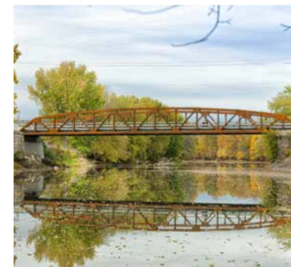
Wynkoop Rd bridge in Hurley.
