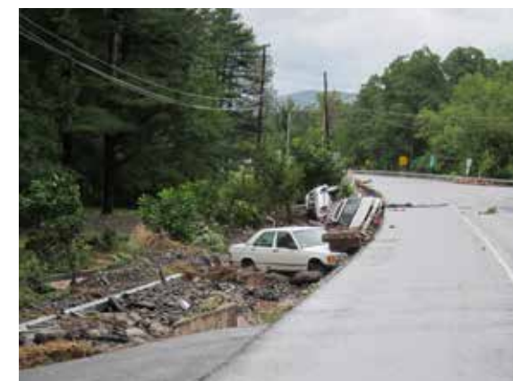
Example of severe flooding and resulting infrastructure and property impacts.
