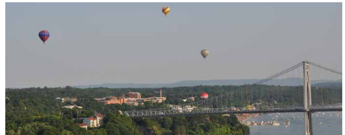
The Mid Hudson Valley Bridge.
