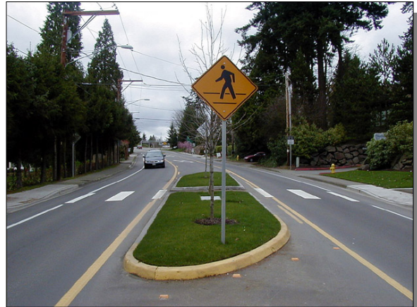
Simple engineering measures such as pedestrian refuges can improve real and perceived safety.
