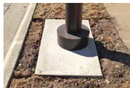
Acceptable Footer Detail
