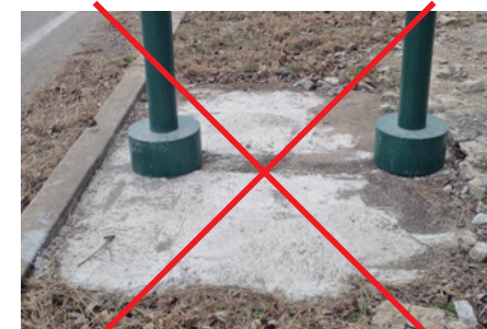
NOT Acceptable Footer Detail
