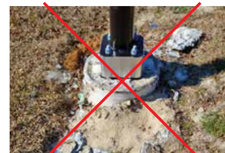
NOT Acceptable Footer Detail
