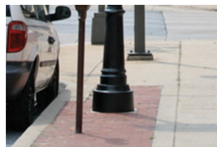
Acceptable Footer Detail
