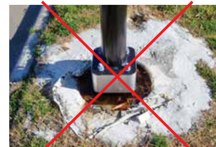
NOT Acceptable Footer Detail
