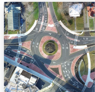
The I587 Roundabout at Broadway and Albany Ave. in Kingston completed in 2022 was designed in part to address congestion in the MHV TMA
