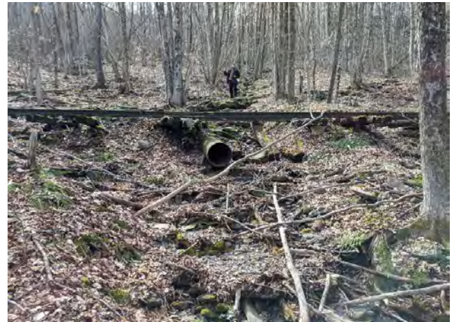
Figure 1-8: Washout just East of Winding Mountain Road (left) and large washout at milepost K38 (right).
