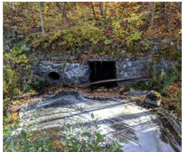
Figure 1-6: Collapsed southern culvert with repair attempts and flowing water visible (left) and inlet of double barrel culverts flowing under railroad (right).
