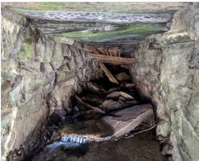
Figure 1-6: Collapsed southern culvert with repair attempts and flowing water visible (left) and inlet of double barrel culverts flowing under railroad (right).
