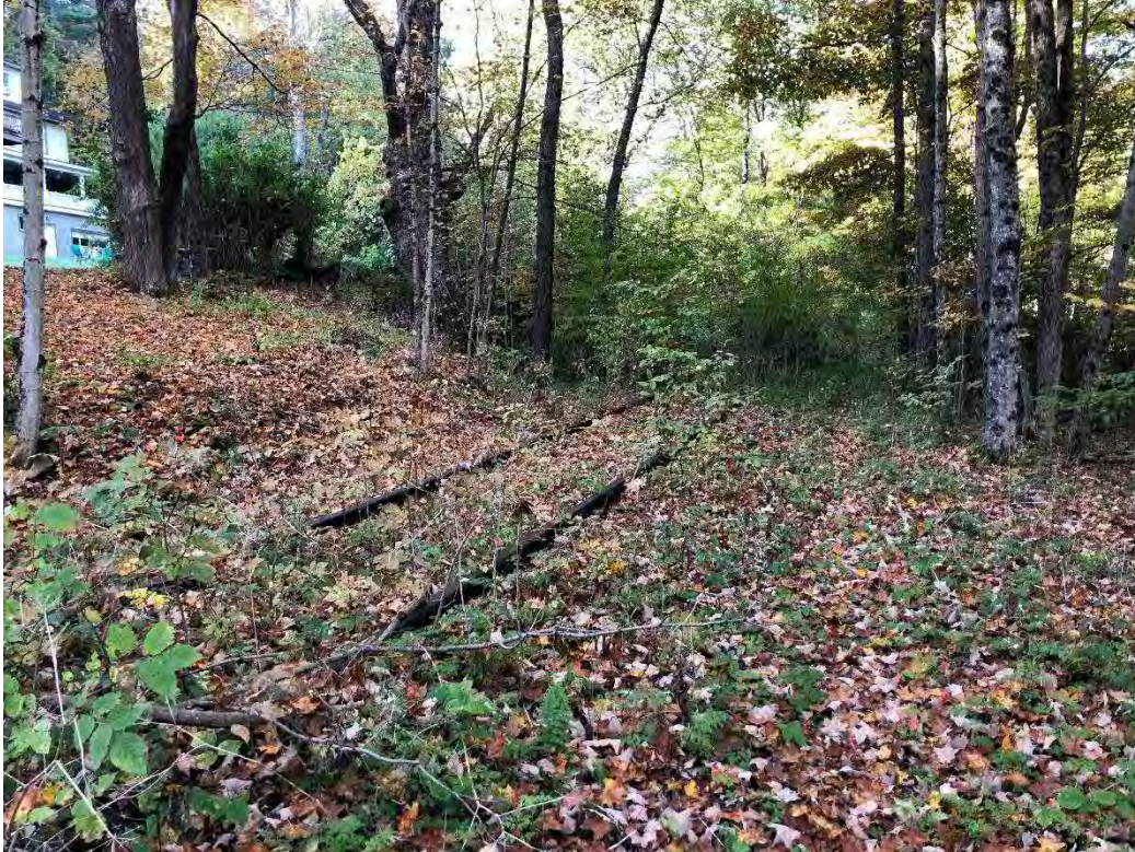
Photo 6. Existing abandoned rail.
