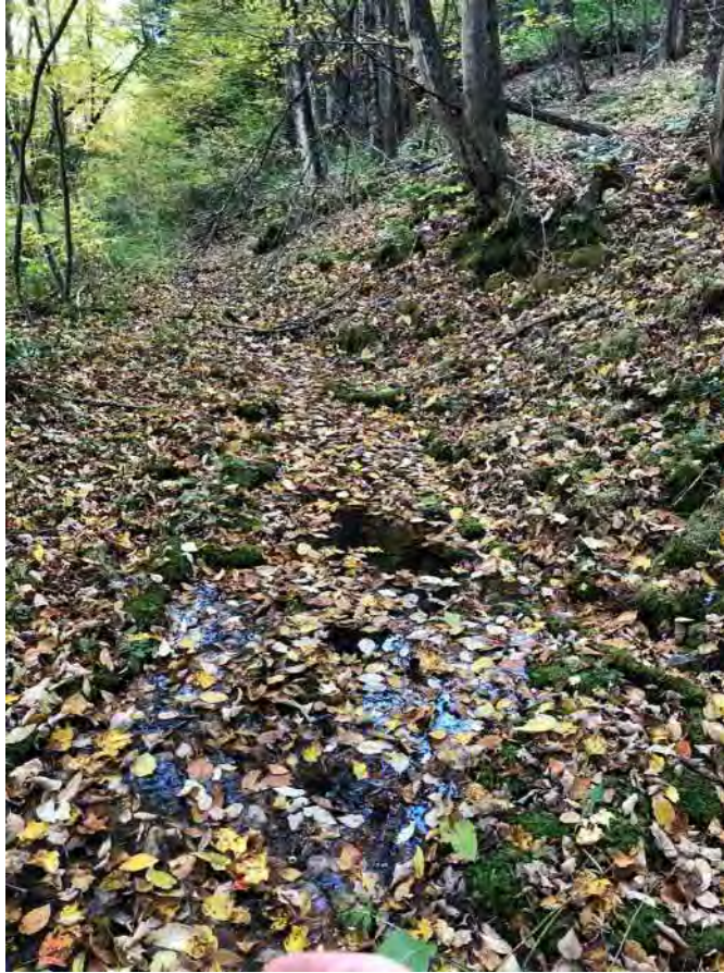
Photo 37. Stream 6 looking north from culvert outlet.
