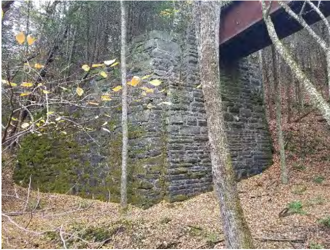
Figure 2-6: Giggie Hollow Bridge East Abutment
