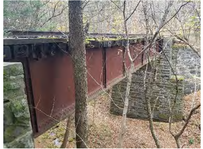
Figure 2-7: Superstructure, looking toward West Abutment
