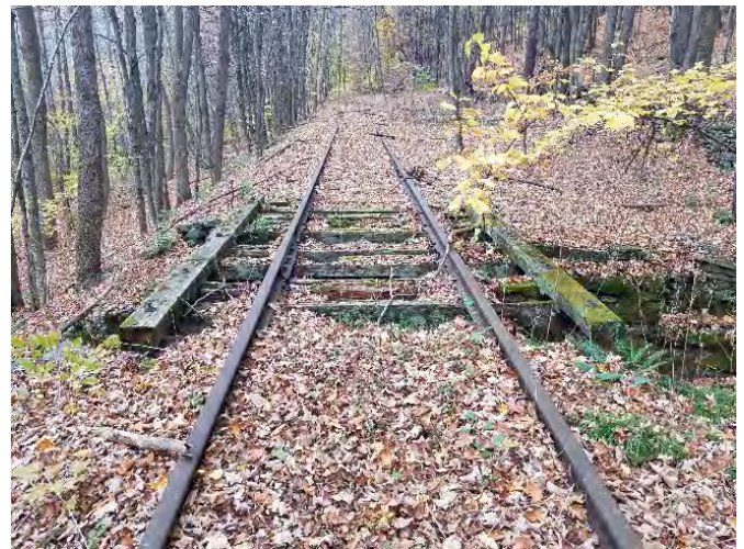
Figure 2-10: Elevation view of Short Span Structure #1
