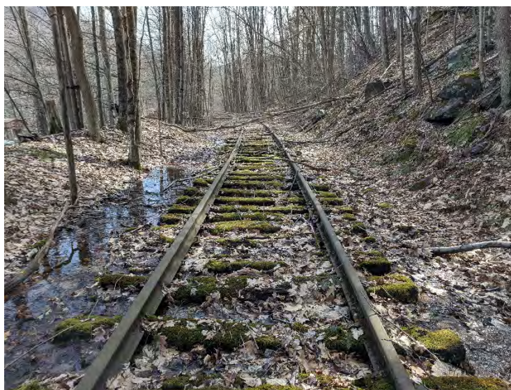
Figure 1-10: Uncontrolled stream just west of Lasher Road.
