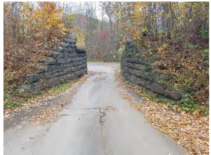
Figure 2 12: Elevation view, showing non-standard horizontal clearance
