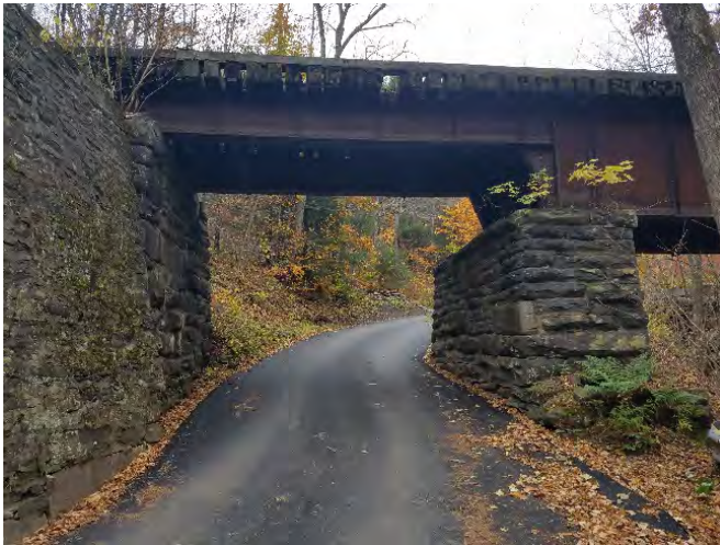
Figure 2-2: Elevation view of Woodchuck Hollow Bridge, Span 1
