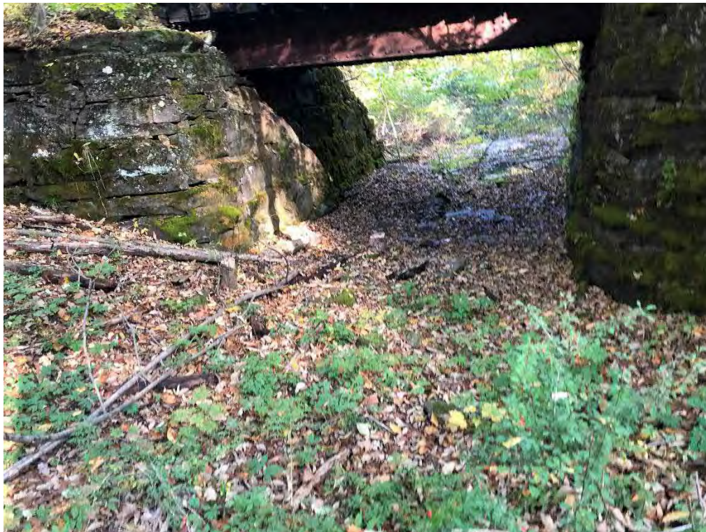
Photo 8. Old cattle crossing/access road. Water is pooled 20 feet north of structure in depression – no stream features or hydrologic connections observed.
