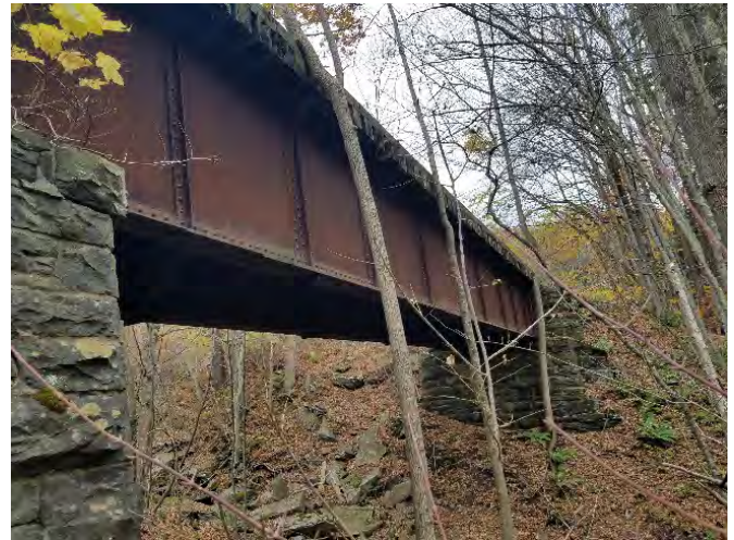
Figure 2-3: View of Span 2 looking toward the West Abutment looking south
