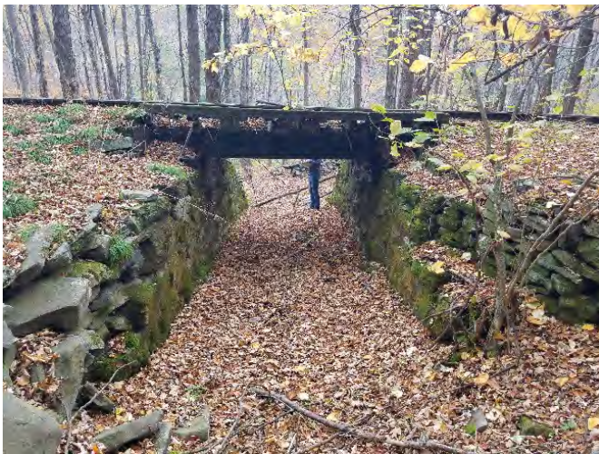
Figure 2-9: View of the rails across the structure, looking south
