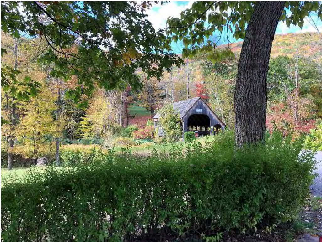
Photo 12. Covered bridge accessing Bellayre Day Use Area over Stream 7.
