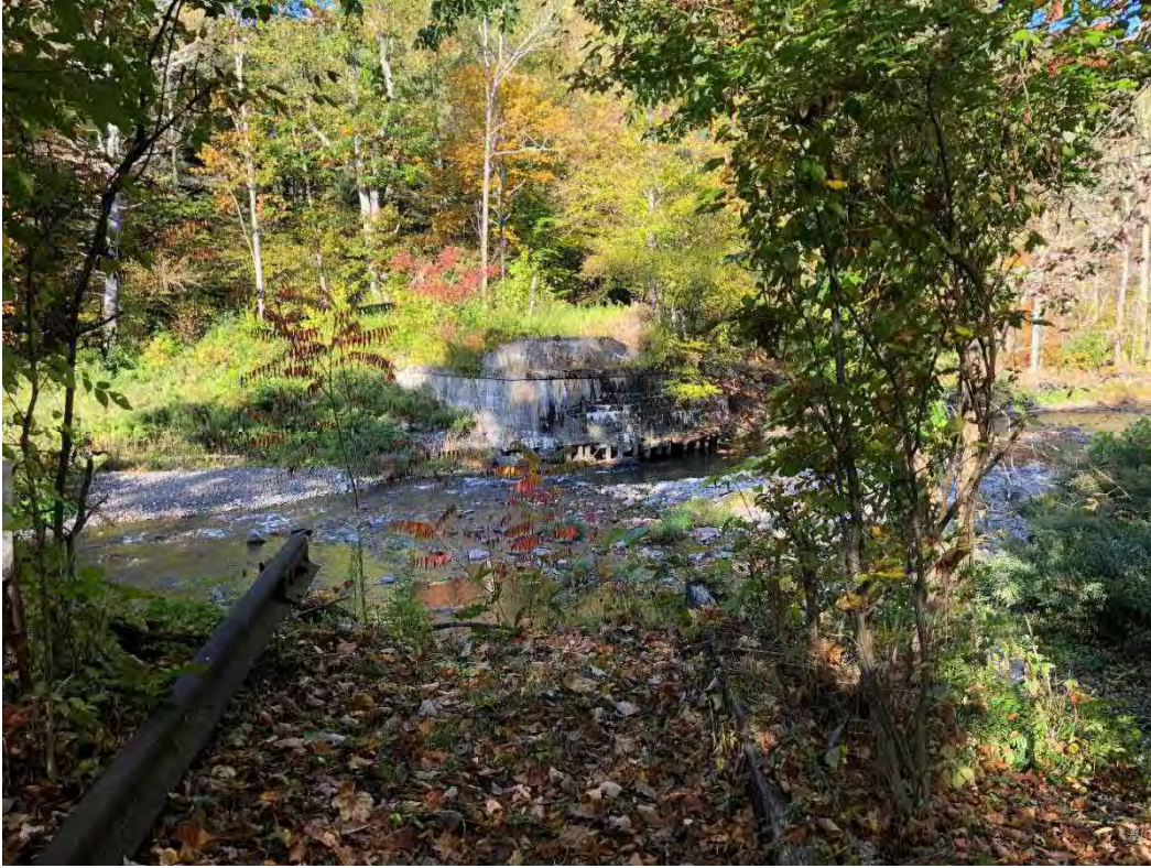
Photo 9. Esopus Creek bridge crossing; structure to be replaced.
