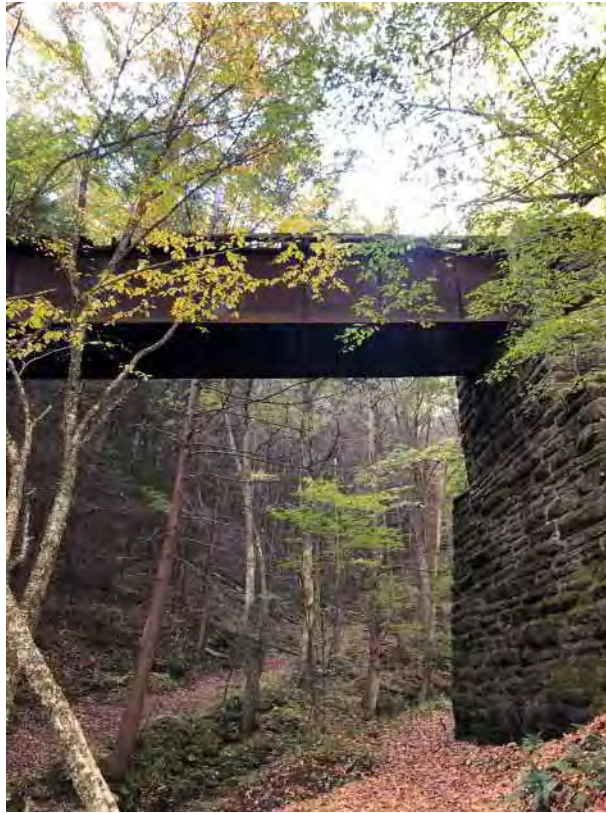
Photo 15. Railroad bridge crossing Giggle Hollow Brook (Stream 8).
