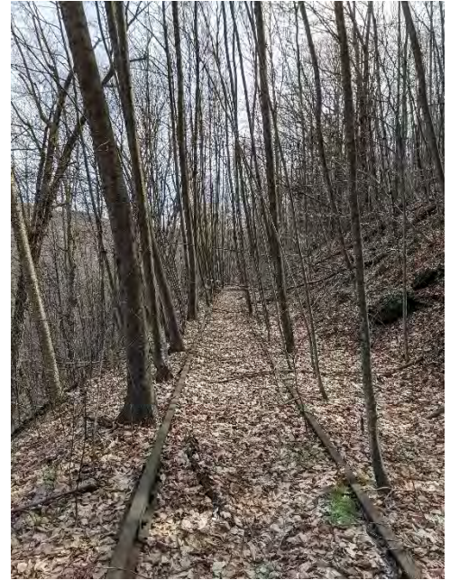
Figure 1-17: Heavy tree growth adjacent to tracks.
