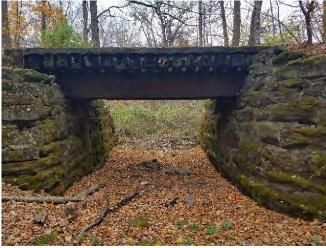
Figure 2-15: Elevation view of Short Span Structure #2
