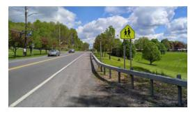
Figure 24: 8-foot shoulder in good condition along Elementary School frontage on 9W northbound, looking north
