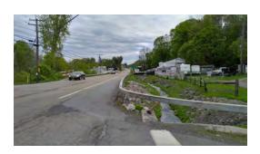
Figure 43: Shoulder in fair condition and guardrail at edge with ditch/creek below on 9W southbound at Perkinsville Road, looking south
