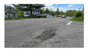
Figure 46: Moderately breaking and cracking pavement in shoulder on 9W northbound at Blue Point Road, looking north
