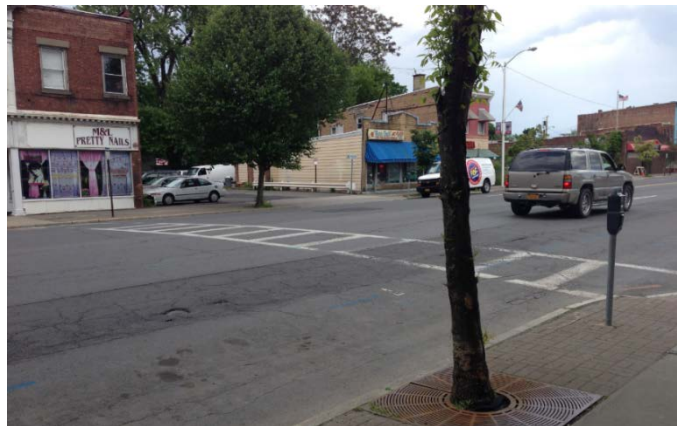
Crosswalk without signs advising motorists
