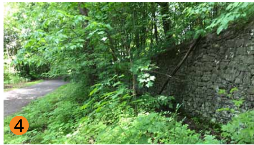
HISTORIC STONE WALL NORTH OF THE STATION, LOOKING NORTH
