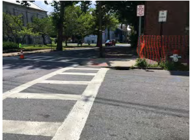
Photograph 2 – Sight distance looking right (D R ) from the north leg of Fair Street
