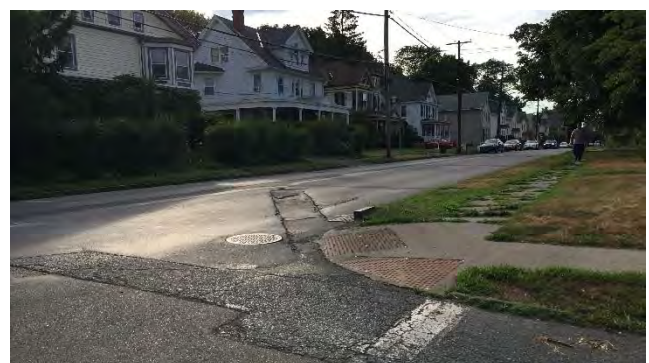
Photograph 2 – Sight distance looking right (D R ) from the east leg of Linderman Avenue
