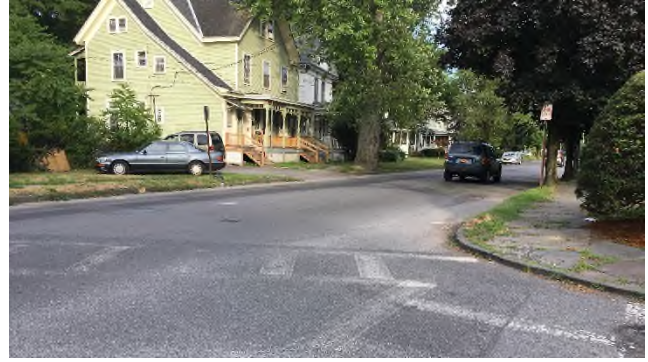
Photograph 4 – Sight distance looking right ( D_R ) from the west leg of Pearl Street
